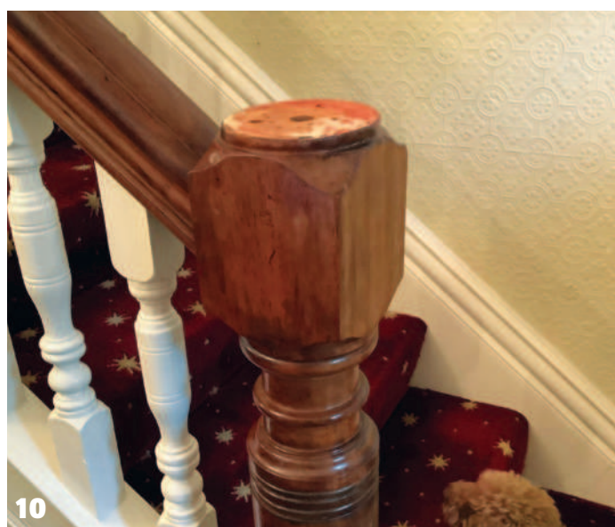
7 Ash doughnut held in my wooden jaws 8 The finished doughnuts 9 My replacement finial 10 The butchered newel post
