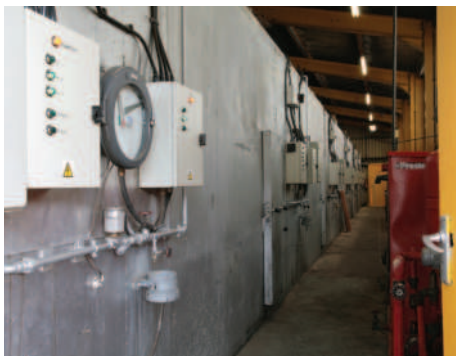
Interior of kiln building
