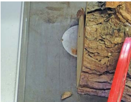
Trimming ends flat
