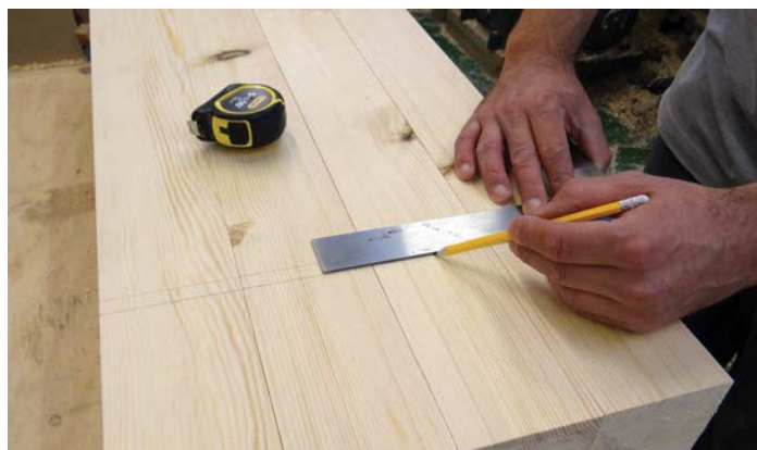
Marking the pommels on the legs all together
