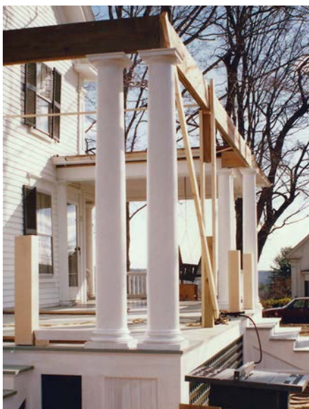
Installing columns at a job site. The blanks are turned from hollow tubes that are coopered from 10 individual staves
