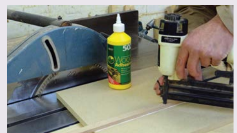
Using my pin gun to hold the batten in place before permanent fixing
