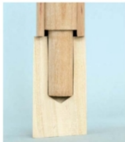
Contacting at the bottom rather than any shoulder, whether present or not, will provide strength and can use the decorative sleeve idea
