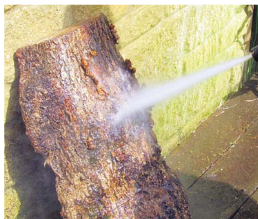
Using a power washer to clean a burr
