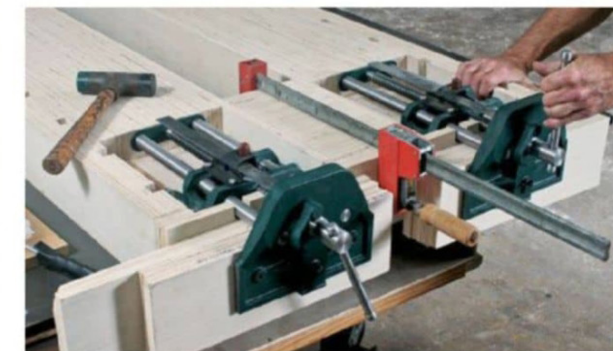
Clamp on the cap. Glue the short end cap over the vises' fixed jaws, using a single clamp and the vises themselves fitted with scrap plywood to clamp the cap tight to the end of the bench.
