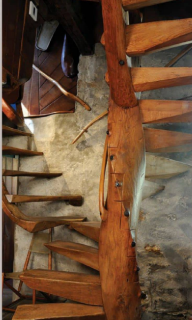
Spectacular steps. Each bolt in Esherick's spiral stair extends through a rectangular cover plate, meeting up with a captive nut in a tread tenon.
