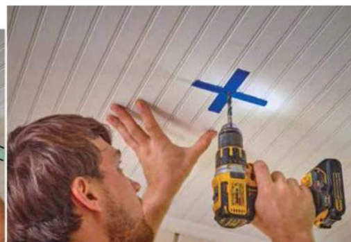
X marks the spots. When drilling pilot holes into the joists I prefer using a bit that's slightly smaller than the diameter of the bolt's shank.
