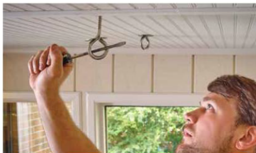
Find the joists. Use a stud finder to locate the joist's center. If need be, you can position the bolts wider than the seat.
