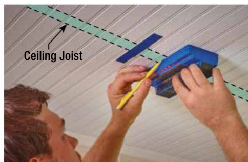
Find the joists. Use a stud finder to locate the joist's center. If need be, you can position the bolts wider than the seat.
