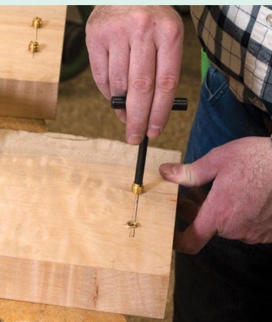
Making a final connection. Loosely bolt both top sections to the leg assemblies, set the glass in the rabbet, squeeze the top together, and then tighten the bolts.
