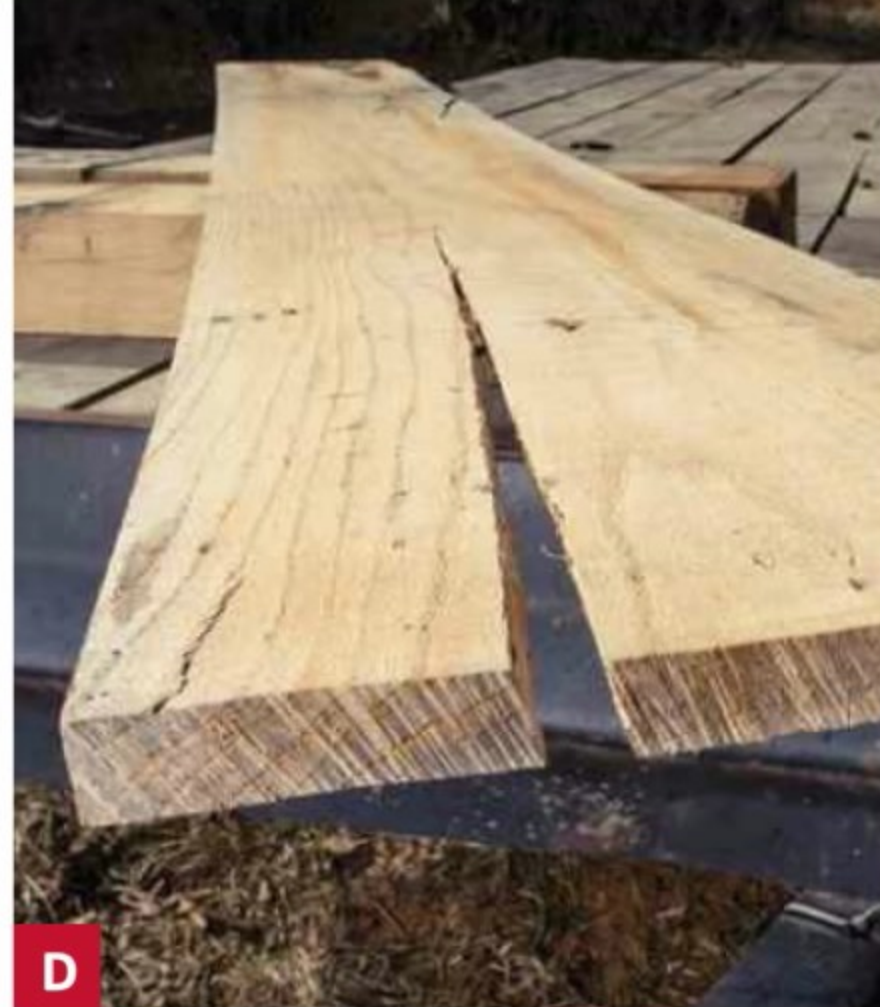
D Board ends crack when they dry out significantly faster than the rest of the board.
