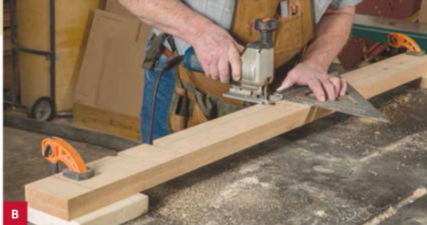
Jigsaw out the waste of the ovals support, cutting towards the holes. Use a rafter square to guide the saw along the crosscut cutlines.
