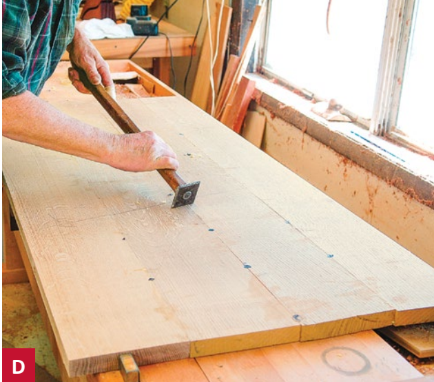
D After the glue congeals and it's safe to remove the clamps, use a scraper to clean up the joints.
