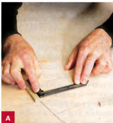
A Set your bevel gauge on the full-scale layout to obtain the exact stave angle.
