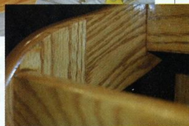
EMLYN JONES USED mortise-and-tenon joinery (see closeup right) for his version of Woodcraft Magazine's Heirloom Quilt Stand.
