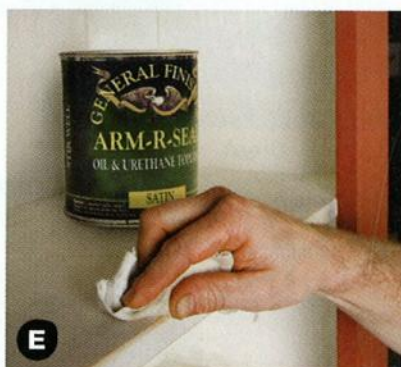
E Use a wiping varnish on the white shelves and cabinet back to seal and protect the paint without adding unwanted color.
