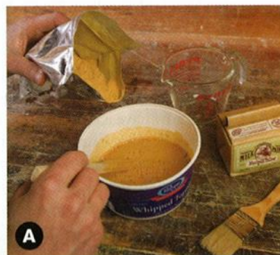
Mix together equal amounts of milk paint powder and water, then gradually add water for better brushing consistency.
