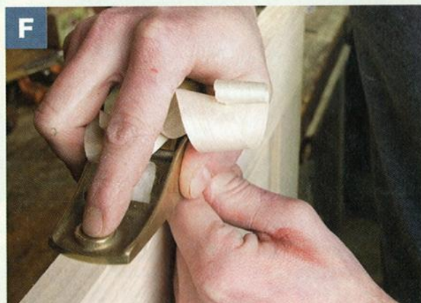
A WELL-TUNED HAND PLANE does a great job on final fitting and creating back-bevels, as well as evening up door faces at joints and door/opening locations.
