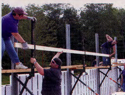
Lie-Nielsen employees, on loan from their respective jobs, recently constructed a new manufacturing facility to meet the demands of the growing tool business.
