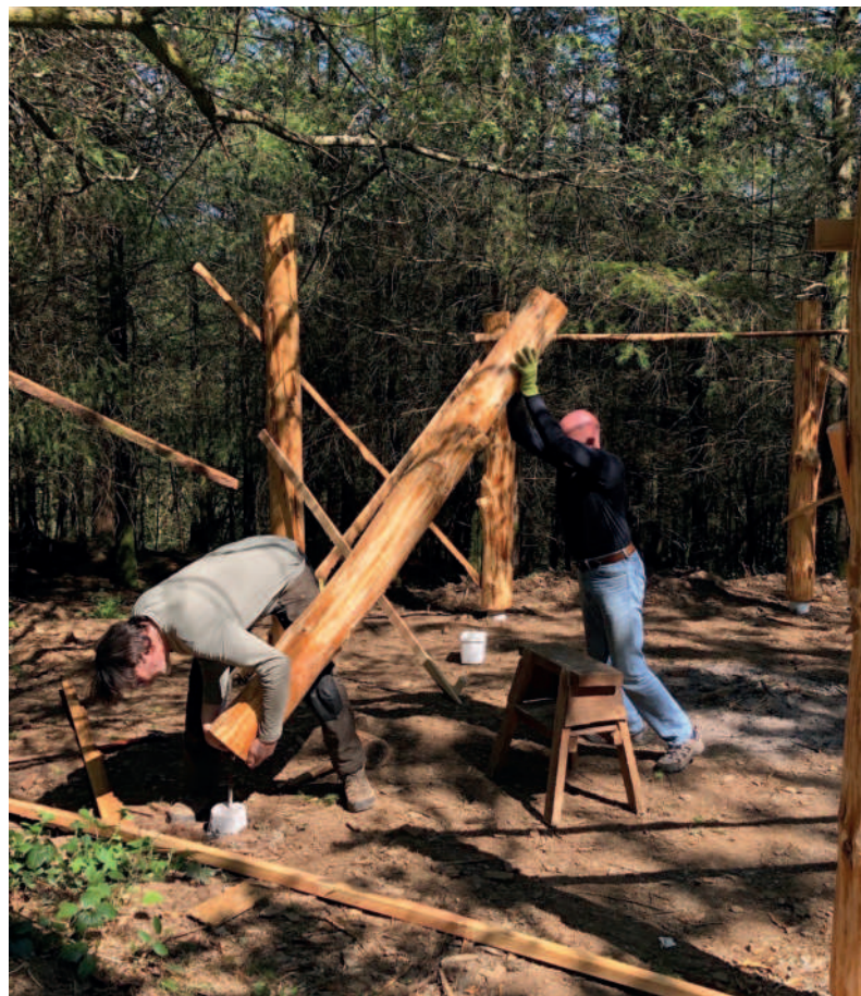
Round house under construction
