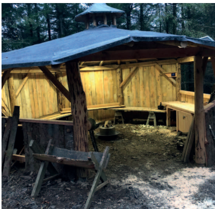
Round house nearing completion
