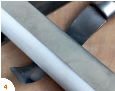
Cleaning up the inside bevel
