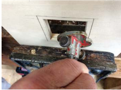
Marking the depth line with a marking gauge
