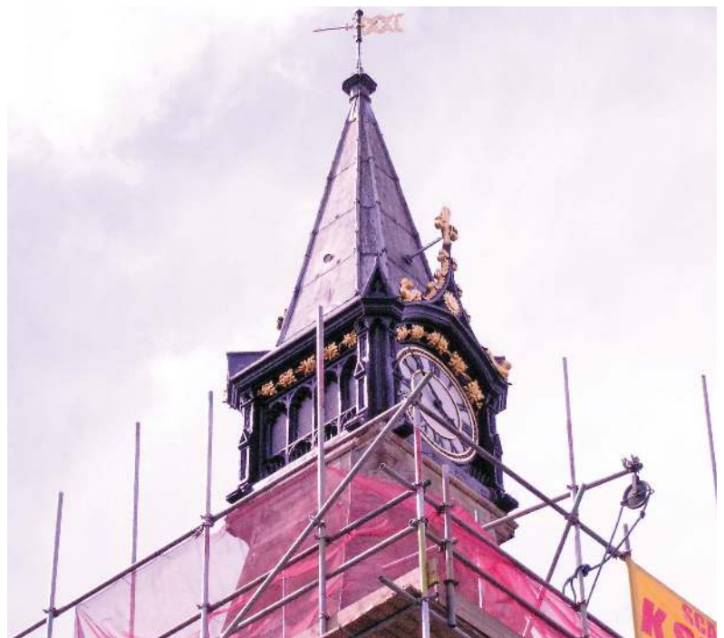
The reconstruction of the Banbury Town Hall clock encasement in the workshop and reinstalled
