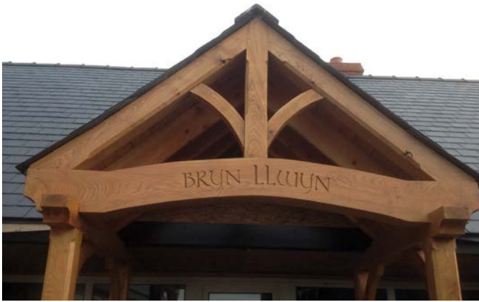
The beam in situ
