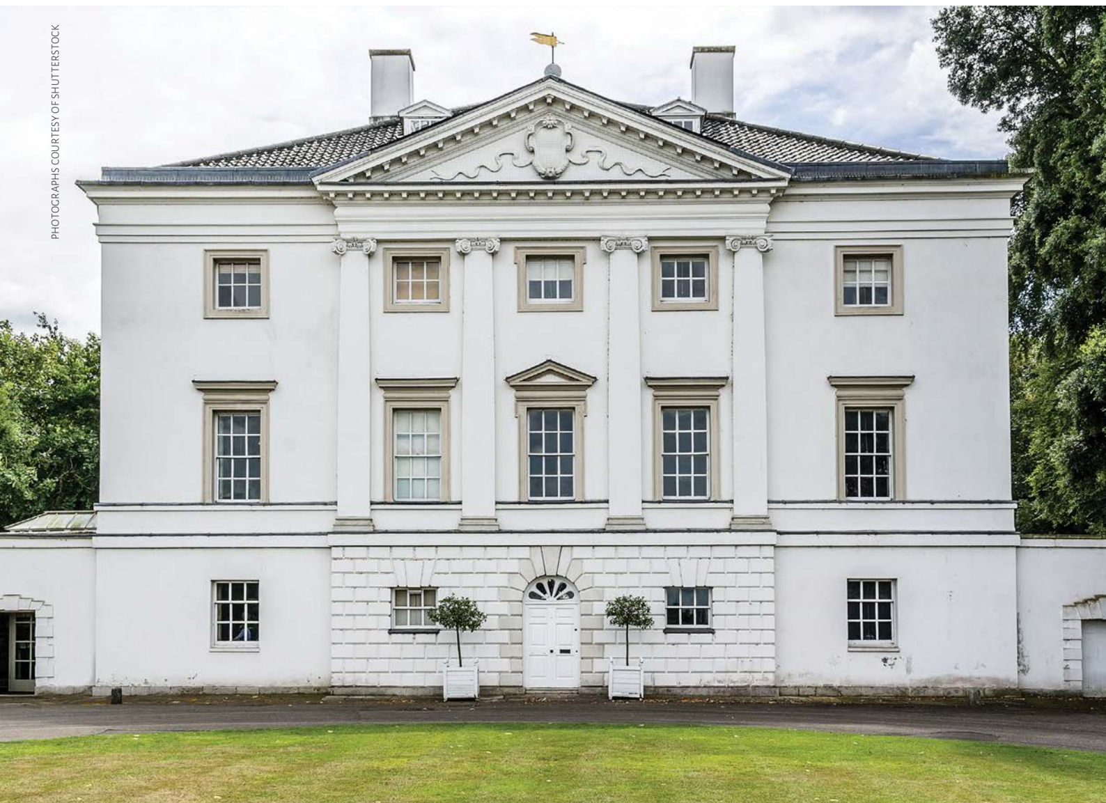
Palladian-style Marble Hill House encapsulates the elegance of the neo-classical Georgian country house
