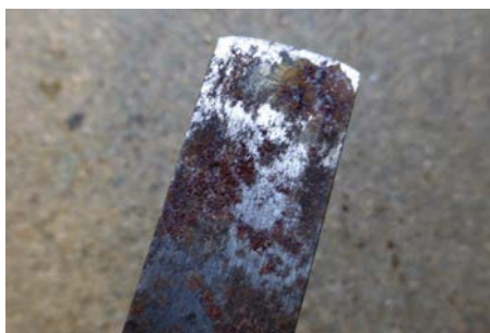
Deep rusted areas are evident
