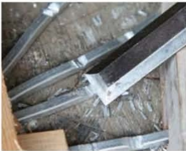
Chopping out 'V' sections with a chisel
