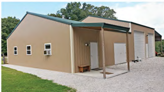
Rick's shop features a resilient metal-sheeting exterior, and double doors that provide easy access for large materials and tools.
