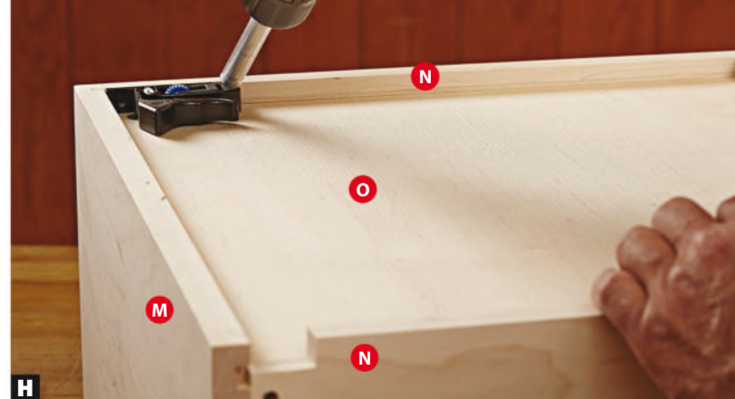
H Position the drawer front clips for your drawer slides. Attach them with furnished screws as directed in the hardware instructions.
