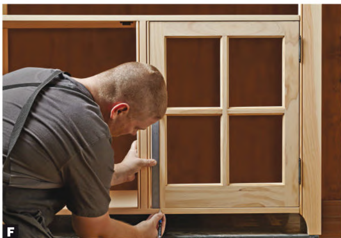
F A rule reveals all. Check for an even gap (reveal) all around the door using a steel rule. With a fine pencil, mark areas that need trimming.
