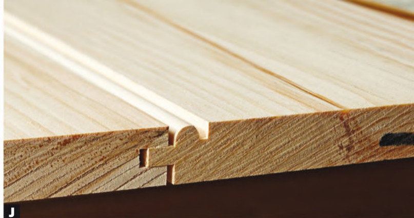
J Create some room to grow. Wood moves across its width as seasonal humidity changes, so you need to leave gaps at every tongue/groove joint so the back slats don't buckle or crack with expansion.
