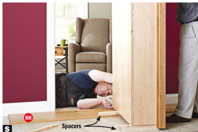
S Position the center case. Have a helper steady the case while you position the turntable and locate the lag screws in the pilot holes.
