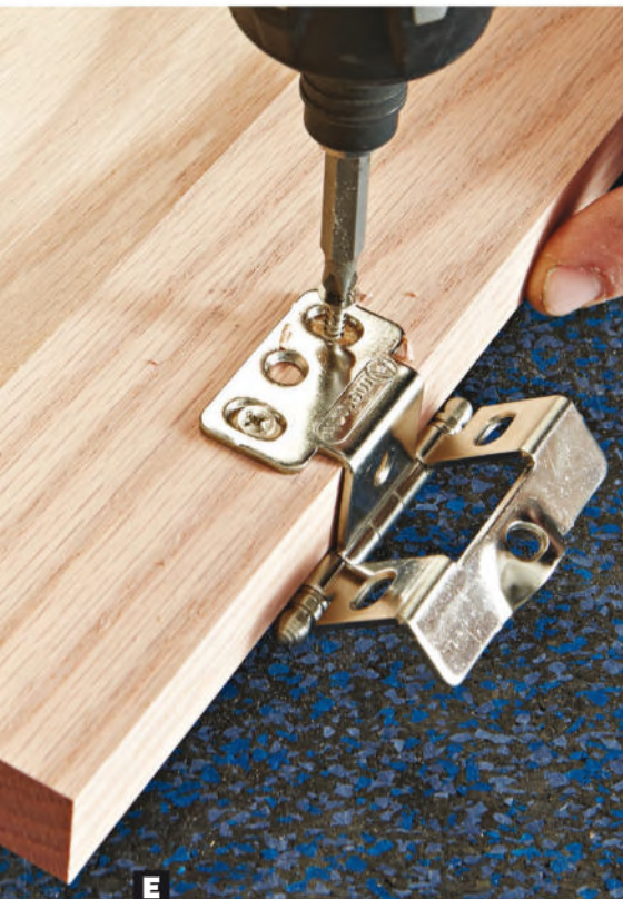
E Shoot for the center. Drive screws in the center of the hinge slots to maximize adjustability. Drill and drive the center screw after making adjustments.
