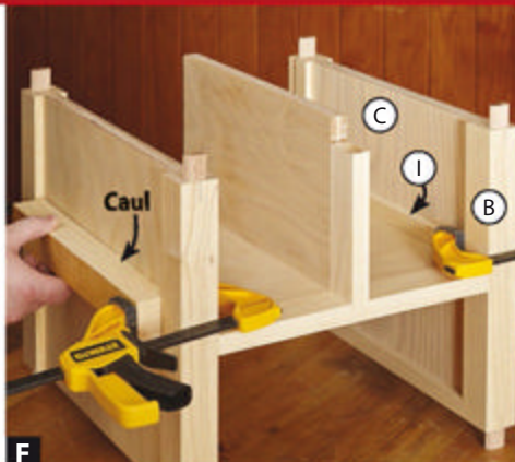
square. After the glue dries, glue on the drawer guides (I) to fill the space between the interior face of the case panel (C) and the edge of the case rails (B). Use cauls
