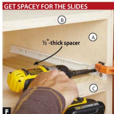
F Rest the drawer slide on a \frac{1}{2} "-thick spacer, aligning the front end of the slide with the edge of the side (A). Screw the slide in place.
