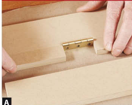
A Capture the hinge leaf with the jig's center strips and side pieces, apply glue to their edges, and clamp them together to make the jig's face.
