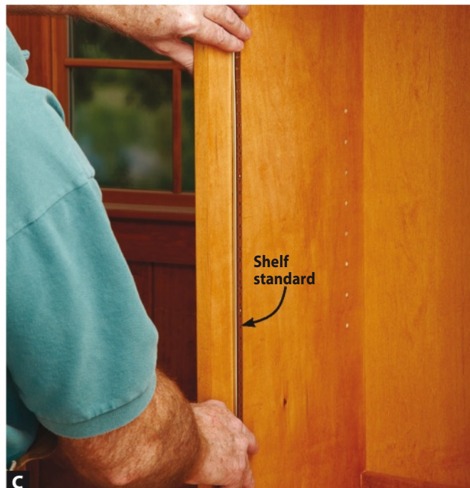
C For best appearance, choose standards as long as the inside height of your bookcase or cabinet. Position screw holes to miss the shelf-pin holes.
