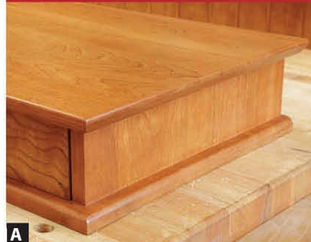
A With the grain direction of the top and side running the same direction, the two panels expand and contract together.
