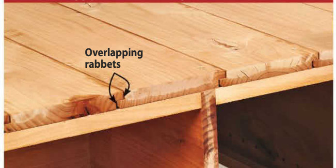
Overlapping rabbets let these boards expand and contract. Applying finish before placing them prevents unstained edges from showing as they move.
