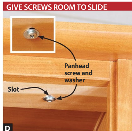
D Elongated screw holes allow room for the screws securing the top of this table to slide within the rails as the top expands and contracts.
