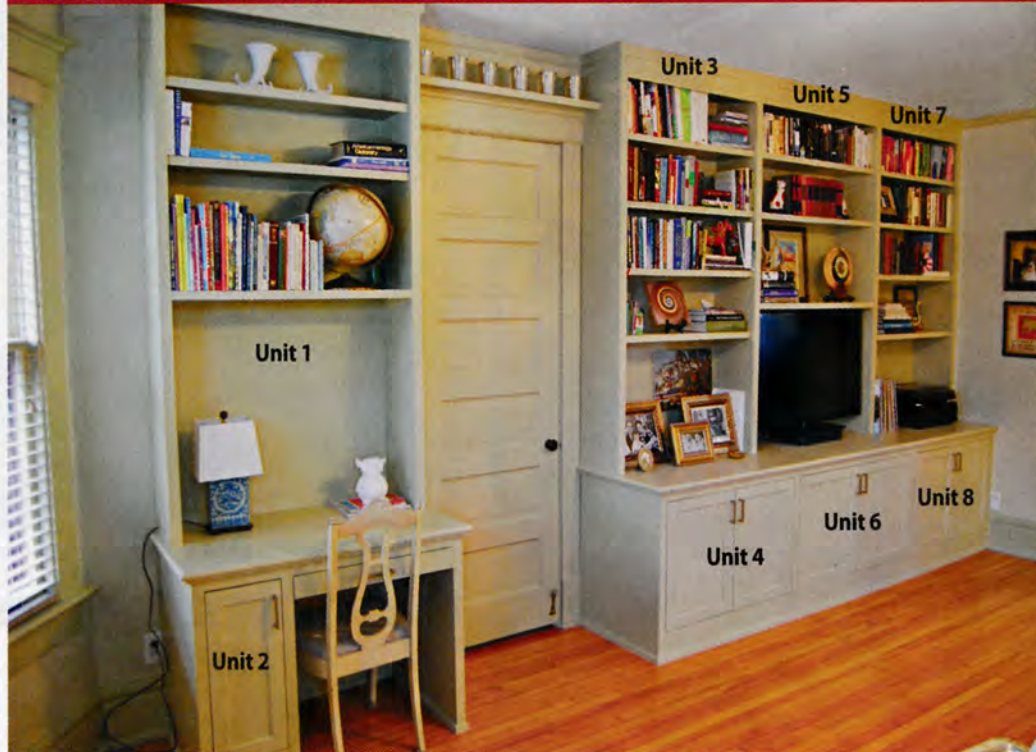
Nelson constructed this floor-to-ceiling built-in in eight units to enable delivery through a small entryway as well as onsite assembly. Constructed separately as single units, the face frames hide the seams between the carcasses, unifying the separate components.
