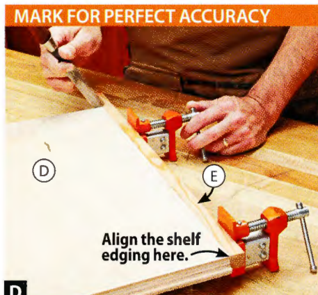
D Align the end of one shelf edging (E) blank with the shoulder of the rabbet and mark the edging's final length with a chisel.
