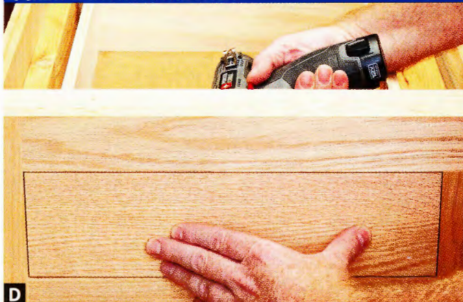
D With the drawer front taped into position with a perfect reveal, provide firm support while you predrill and screw it in place.
