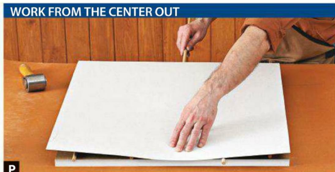
P Beginning in the middle, pull out a dowel while pressing the laminate to the substrate. Remove the dowels to one side, then to the remaining side.
