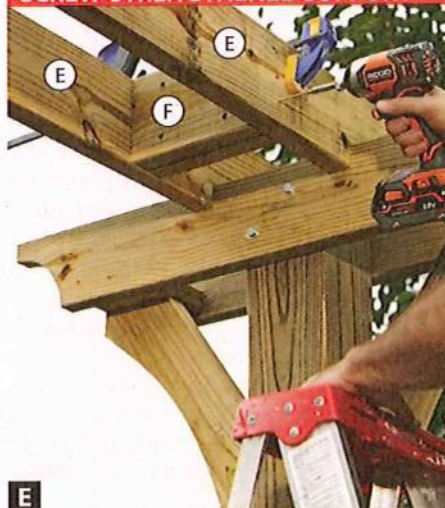
Drive six 3" deck screws into each end of the chain blocking (F/F), offsetting them to avoid the screws within the blocking.
