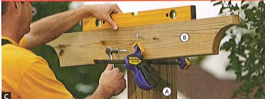
Clamp a cross beam (B) flush with the top of the post (A). Drive one lag screw. Level the cross beam, and drive the second screw. Repeat with the second cross beam; then add the cross beams to the other post.
