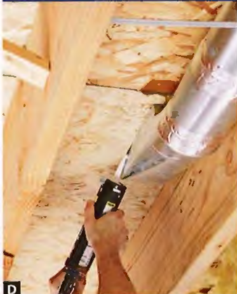
D Seal gaps where heating ducts, water pipes, or other items penetrate walls and ceilings shared with living spaces.
