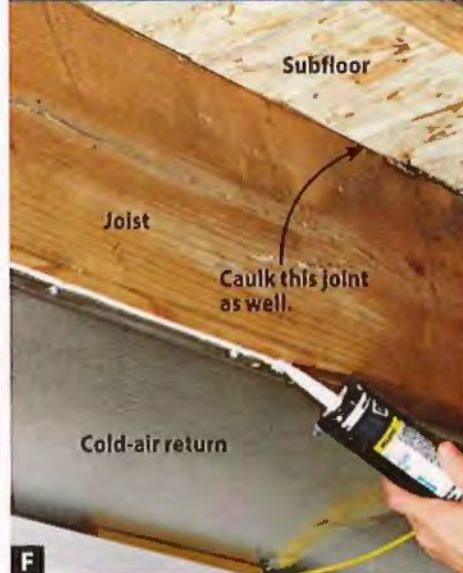
F Caulk the seam where the sheet metal meets the bottom of the joist, and where the top edge of the joist meets the subfloor.
