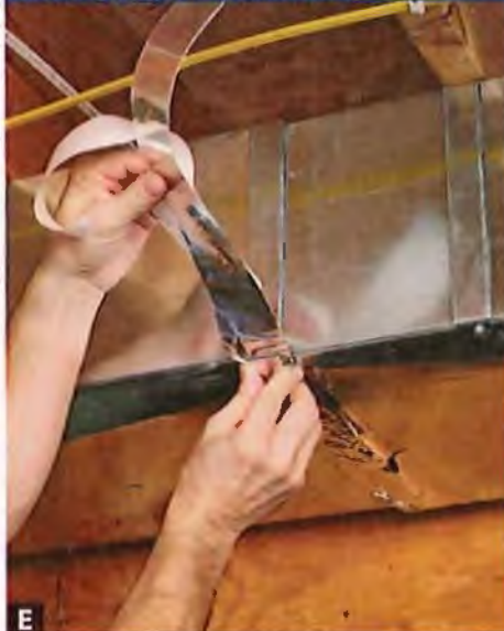
E Apply self-adhesive foil tape along joints in duct-work. Wipe the duct clean so the tape sticks, and smooth the edges to the metal.
