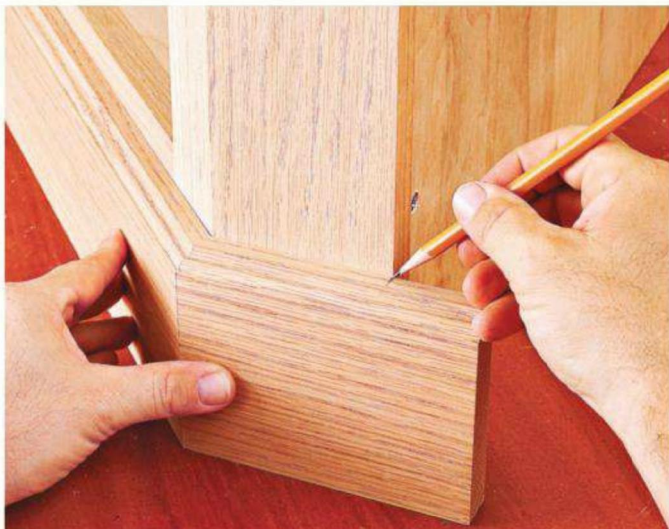
Test and perfect the angle of the miter on an oversized blank before marking and cutting the trim piece to the final length.
