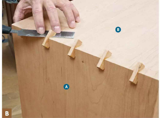
Use a flush-cut saw to cut both ends of each key flush with the case. Then, finish-sand the outside of the case.
