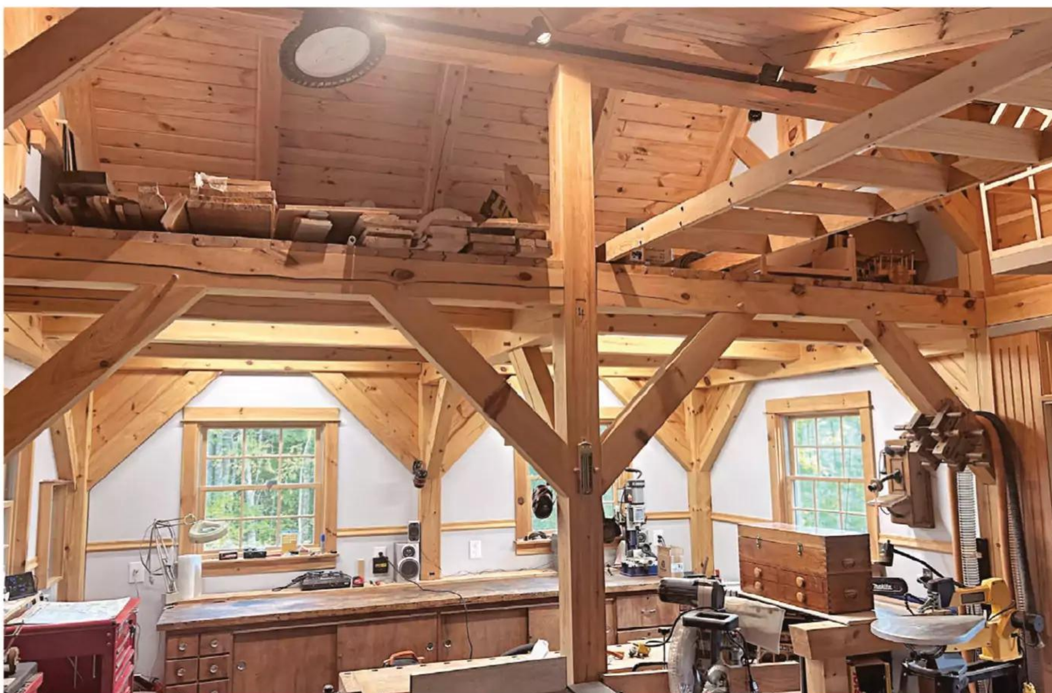
A loft with tongue-and-groove flooring offers an ideal storage space for lumber. The custom ladder raises and lowers using a rope and pulley system Bob designed.
