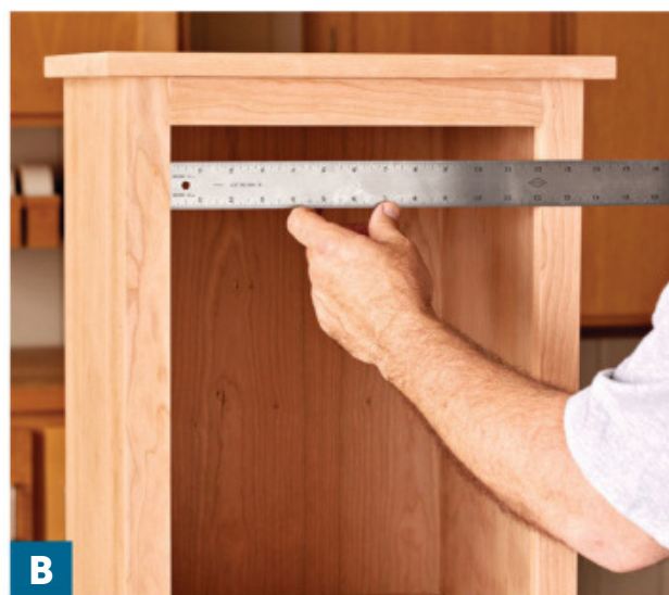
B Measure the width and height of the opening at several points. Use the largest measurement in each direction when sizing your door.
