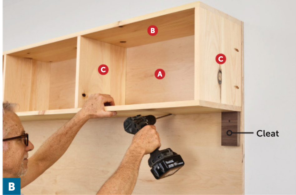
B Position the cleats to place the top of the shelf assembly flush with the top of the backer (A). A helper may be needed to steady the shelf as you drive the pocket screws.
