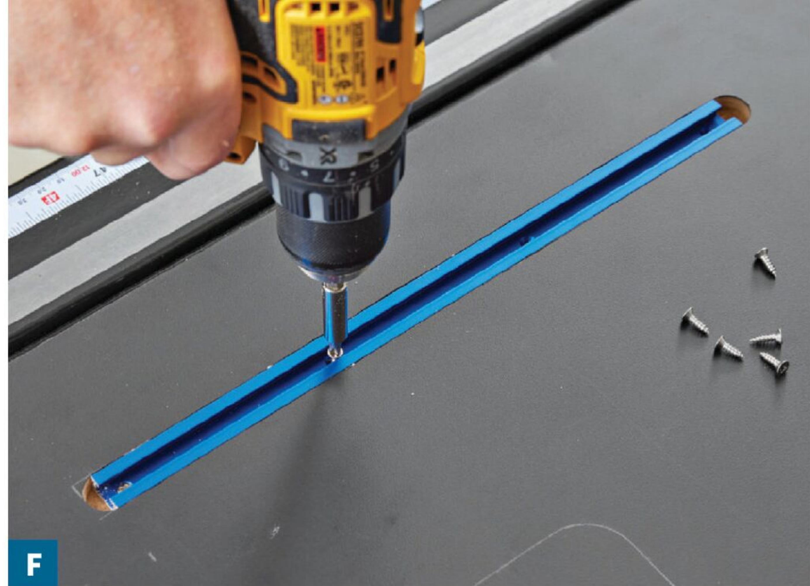
F Center the T-tracks in the length of the slots. This allows space for the bolts that hold the fence to drop in and engage the track. Secure the tracks using short screws.
