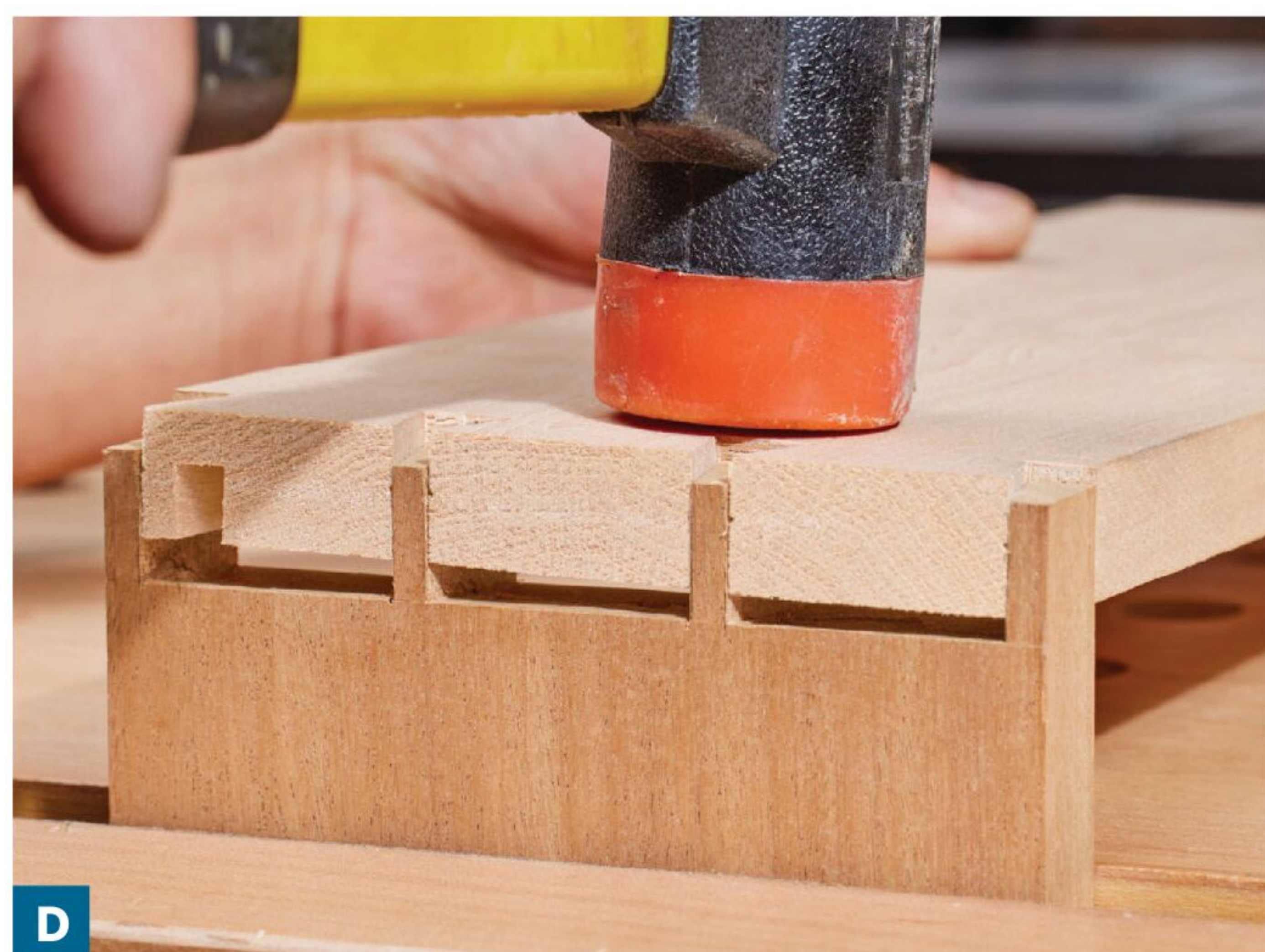
D Dry-assemble the drawer to ensure the joints are tight and the sides are square.
