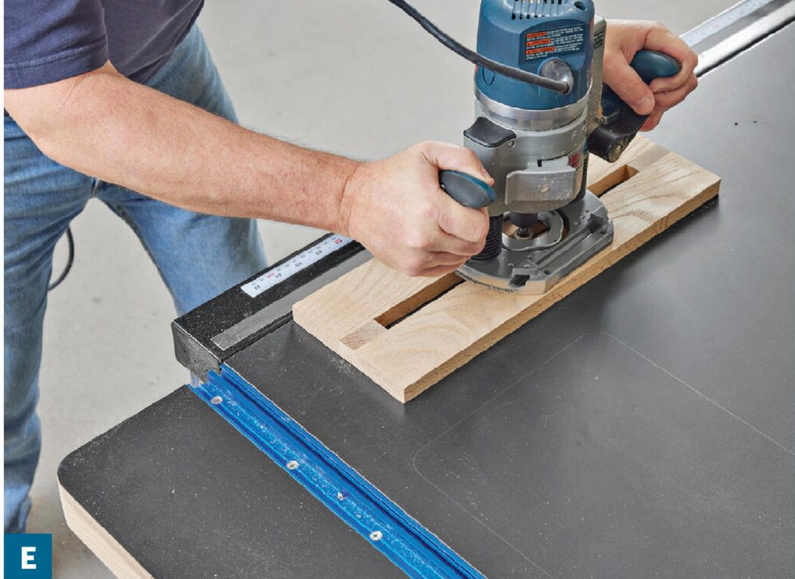
E Position the T-track guides on the table so they'll align with mounting slots in your router-table fence, securing them with double-faced tape. Rout the slots using a dado-cleanout bit.
