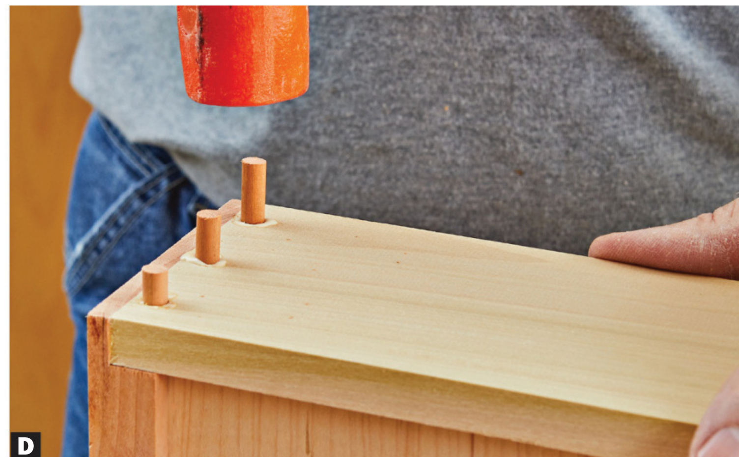
D Glue dowels into the holes. Cut them flush when dry, then sand smooth.
