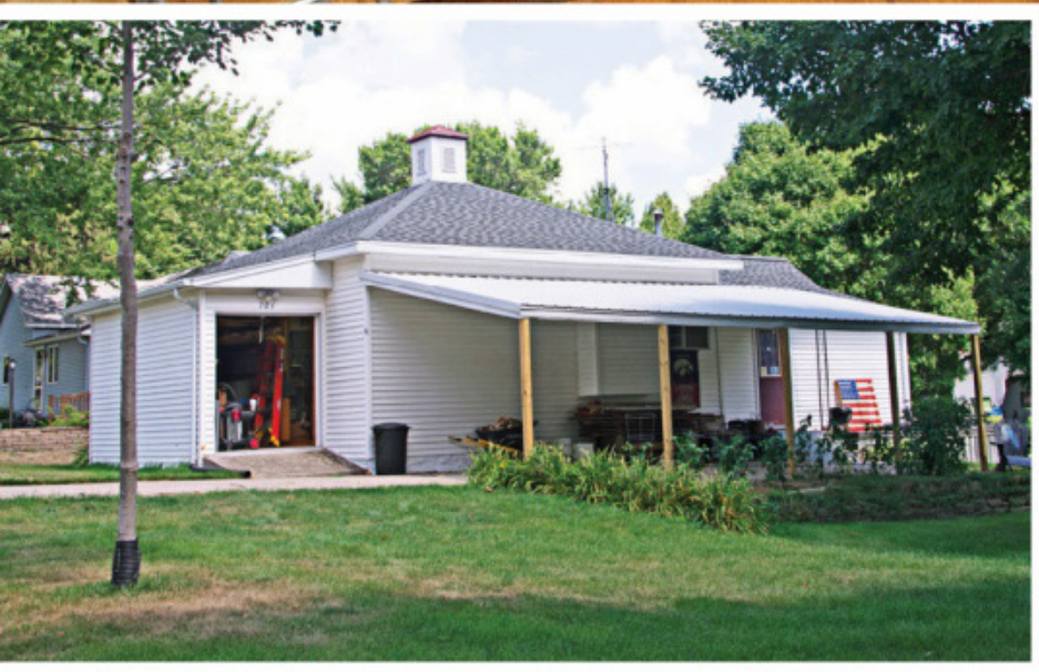
Bud Bieker's workshop, once a church, now sports a cupola rather than a steeple.
