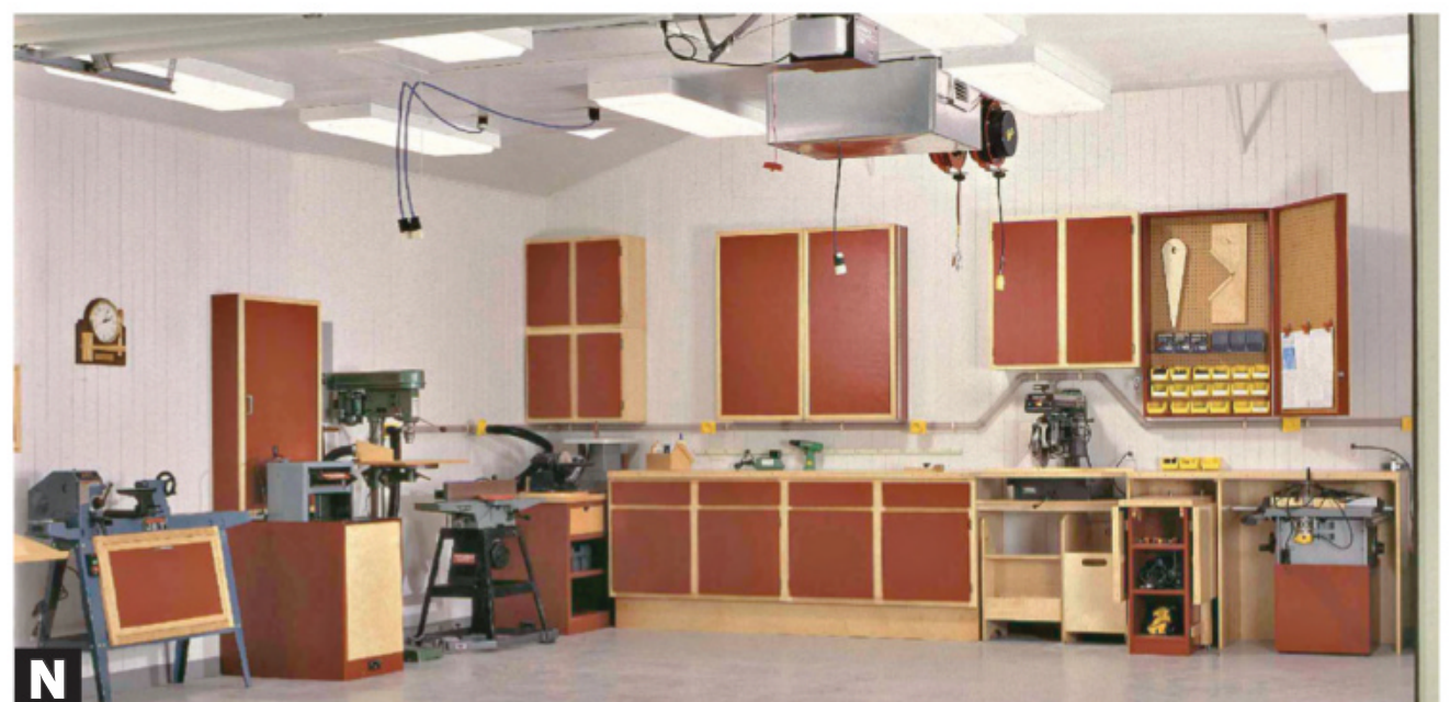
M A collector mounted in the rafters frees up shop space, allows overhead ductwork, and reduces noise. Just make sure you have access for emptying the bin or bag.
