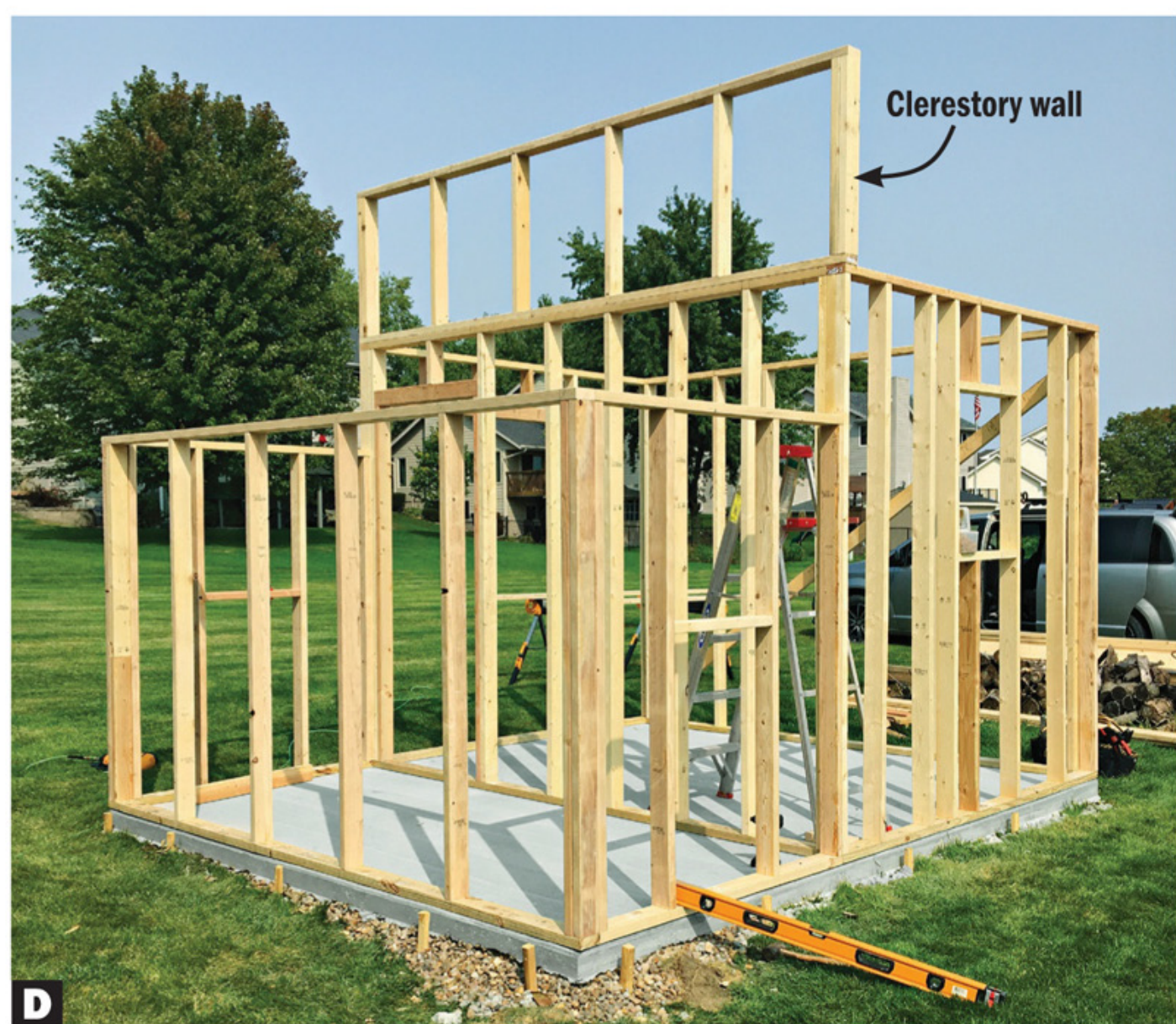
D Assemble the clerestory wall on the ground, then enlist the help of an assistant to lift the wall up and set it into place.
