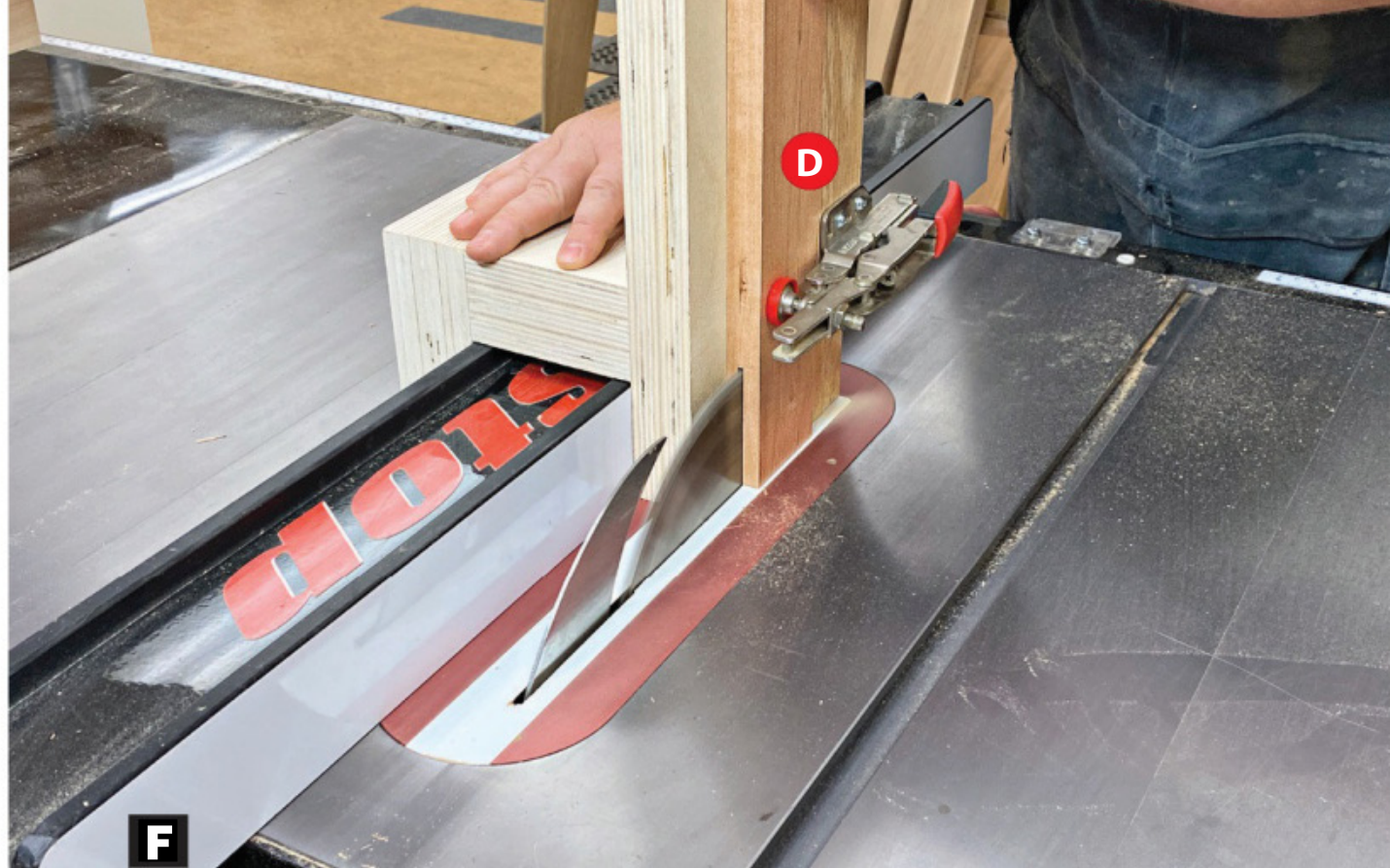
F Position the rip fence to roughly center the blade on the trim. Make a pass on each face, then adjust the rip fence to cut the mortise to finished width.
