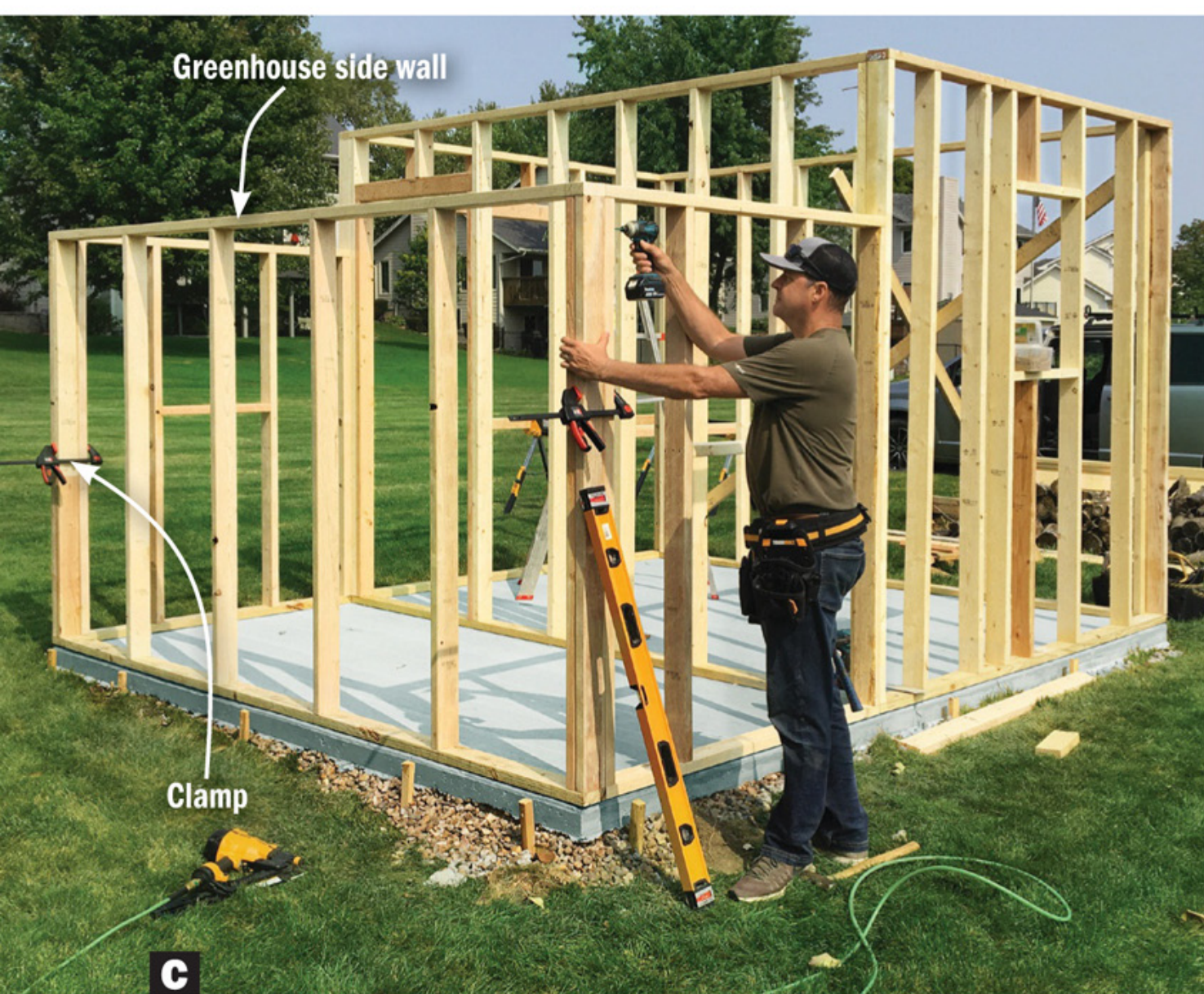
C Clamp the side wall of the greenhouse to the ends of the front and back walls to hold it in place while driving the screws.
