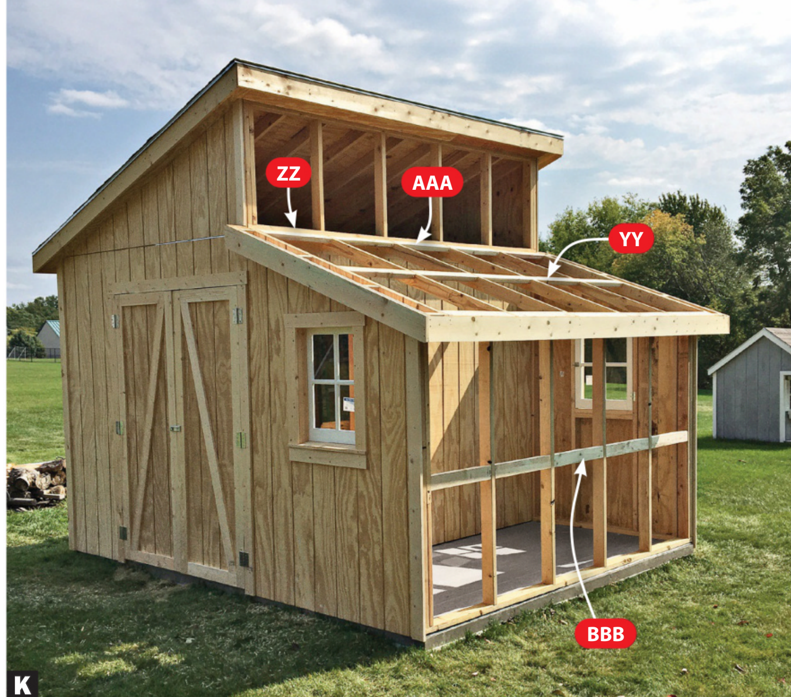
K Purlins (YY) and blocking (ZZ, AAA, BBB) provide support for the polycarbonate roofing panels.
