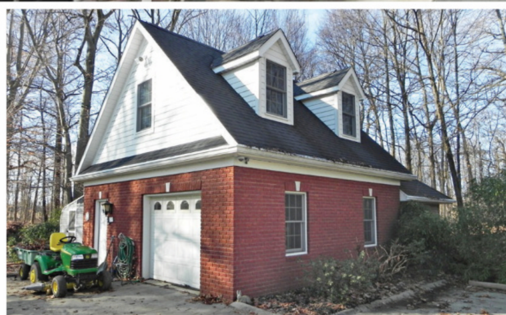
Eric designed his woodshop with an attached greenhouse to support his gardening hobby. The second floor will house an office, exercise area, and finishing room.
